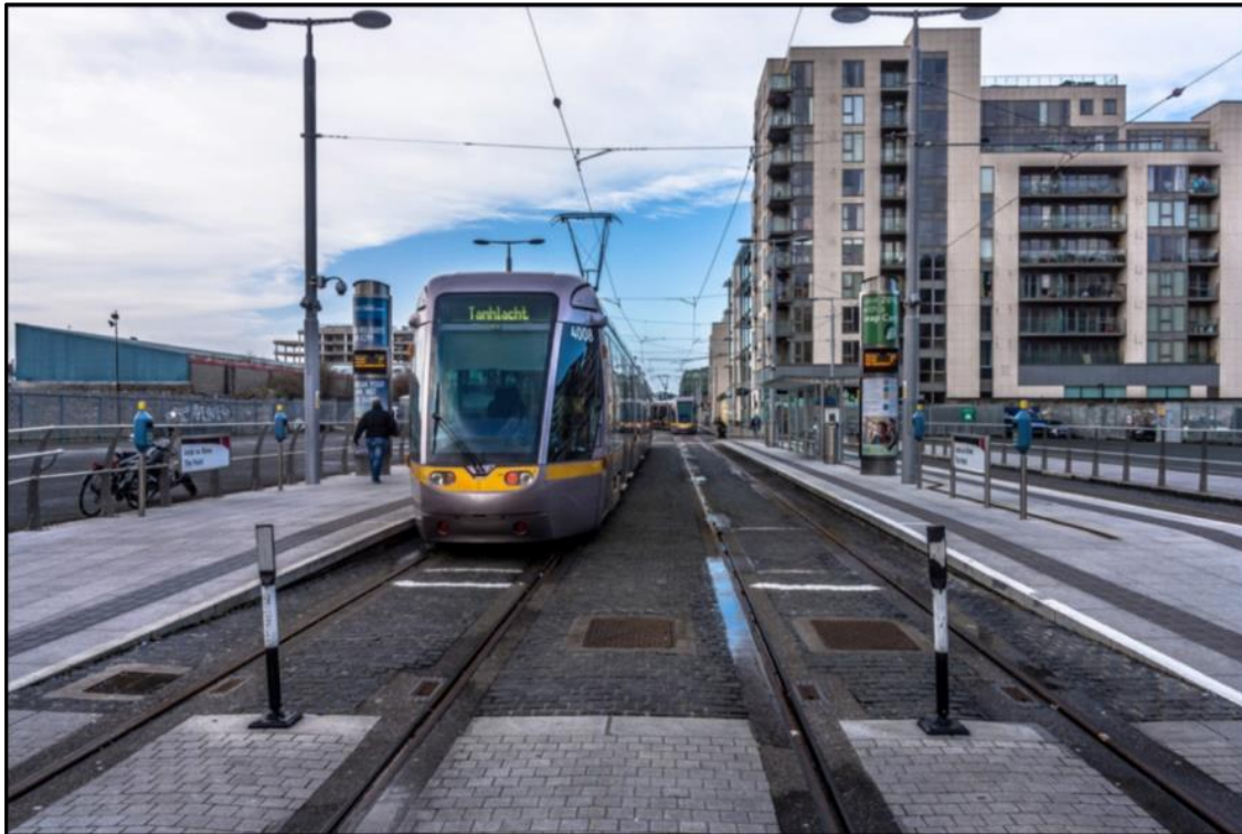
Figure 13-39 Luas Facilities at 'The Point'
