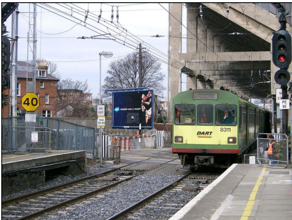
Figure 13-41 Facilities at Lansdowne Road Station
