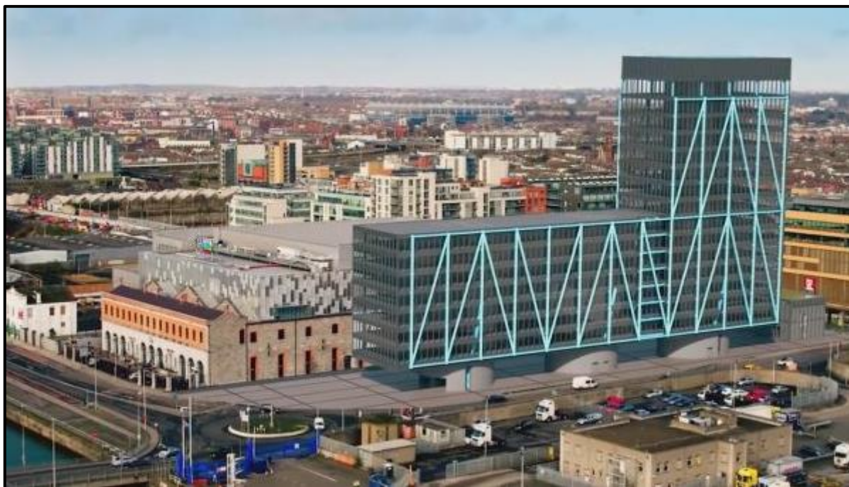
Figure 13-94 Illustration of the Consented Exo Building Currently Under Construction
